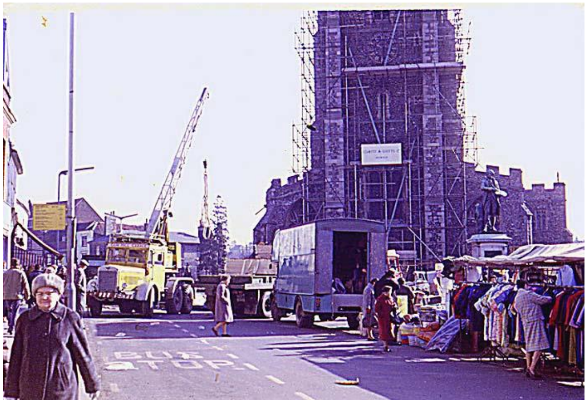
1968 work in progress to remove the spire from St. Peter's
